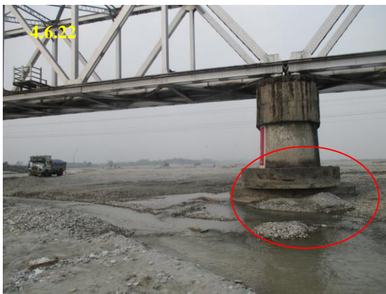
Plate 4.6.22 & 4.6.23 Bed incision at the foot of railway piers.
