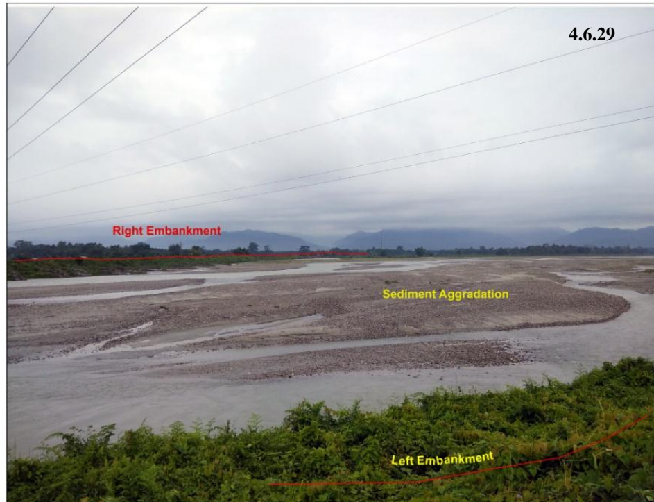
Plate 4.6.29 Copious sediment aggradations forming huge gravel bars in the immediate upstream of railway bridge, Odlabari. Note the least difference in elevation between the river bed and the embankments.
