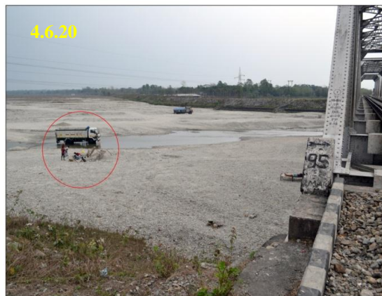
Plate 4.6.20 Sediment mining operating barely 100m upstream of the Odlabari rail bridge; 4.6.21 Sediment mining operating under the Odlabari road bridge.(Photographs taken- 21.03.2013)
