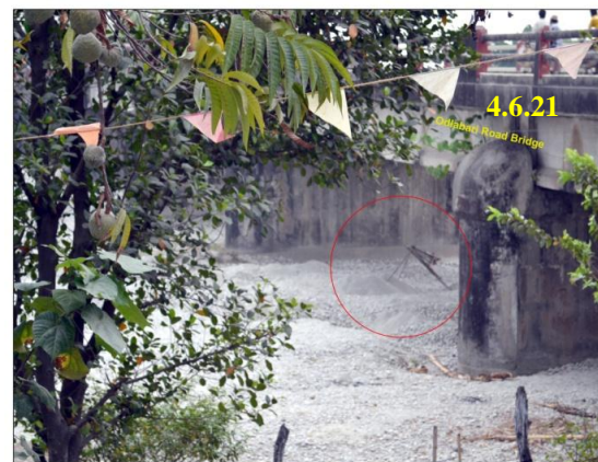
Plate 4.6.20 Sediment mining operating barely 100m upstream of the Odlabari rail bridge; 4.6.21 Sediment mining operating under the Odlabari road bridge.(Photographs taken- 21.03.2013)
