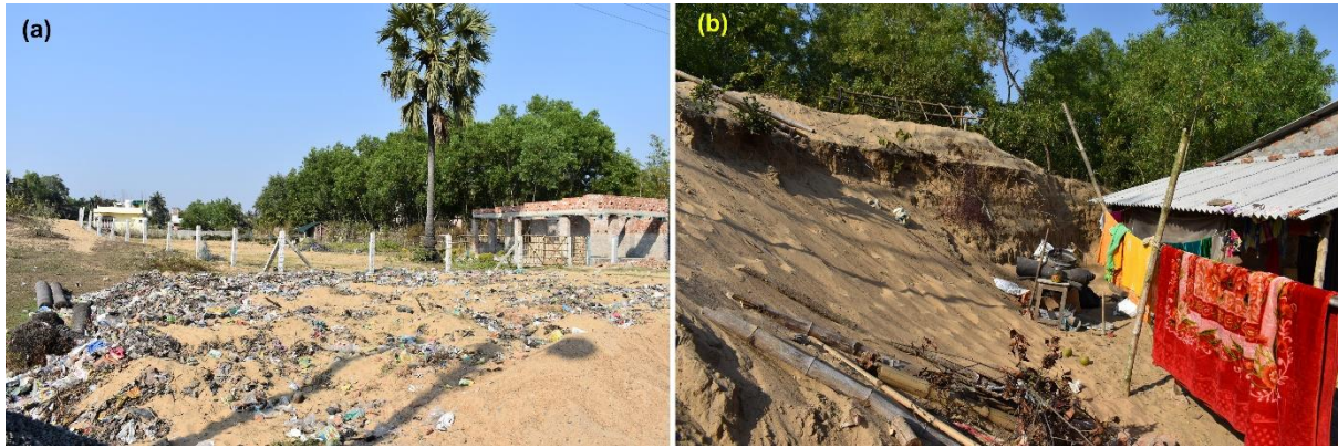
Plate 5.1: Dune cutting (b) and flattening (a) for housing construction in Contai.
