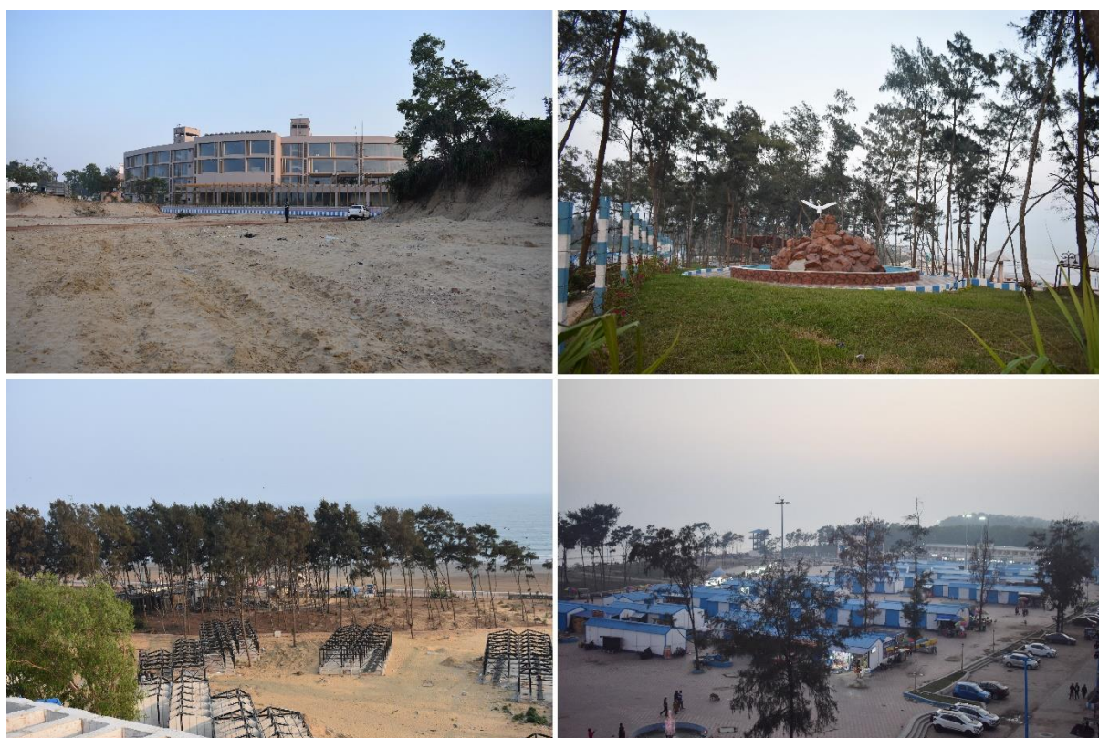
Plate 2.3: Degeneration of dune habitats by the tourism infrastructural development at Digha.
