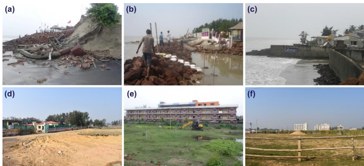
Plate 2.11: Erosion and damages of the hotels by the storm effects at the shorefront areas (a-c) and new hotels are coming up at the backshore areas over the wetlands (d-f) in the Mandarmani coastal stretch.
