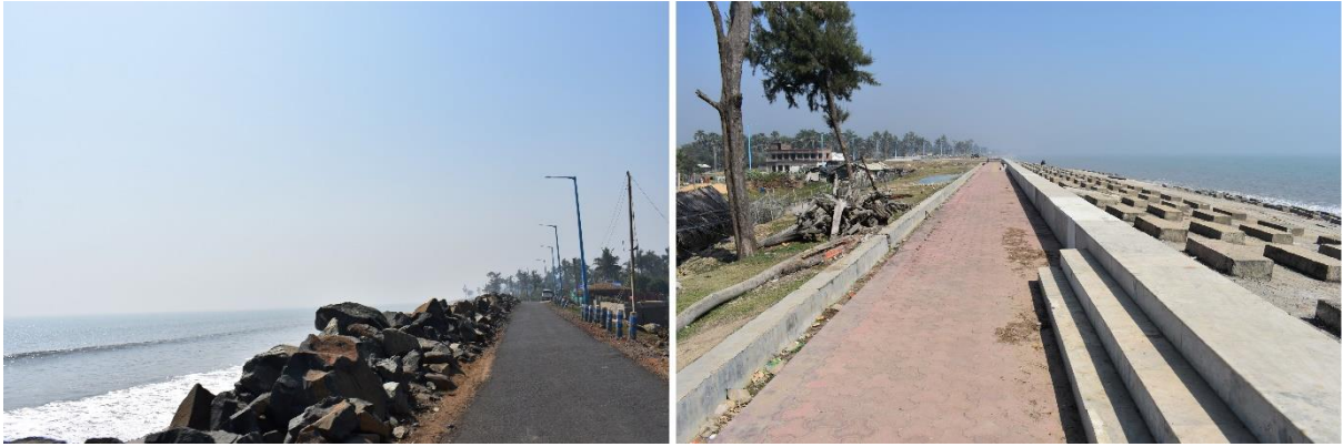
Plate 2.12: Concretization of the shorefront areas at Tajpur-Sankarpur coastal stretch.
