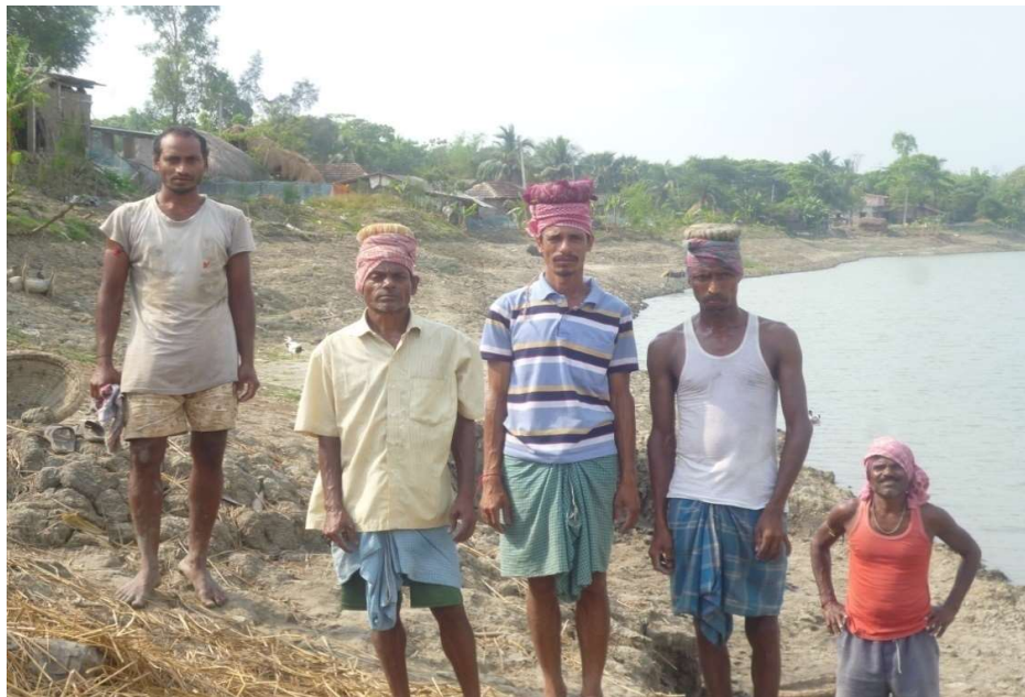
PICTURE-16: LABOURES DOING RENOVATION WORK AT TETULIA KHAL
