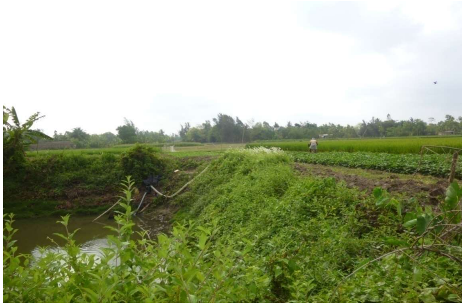
PICTURE-18: A PRIVATE TANK NEED TO BE RENOVATED AT PATHARPRATIMA BLOCK
