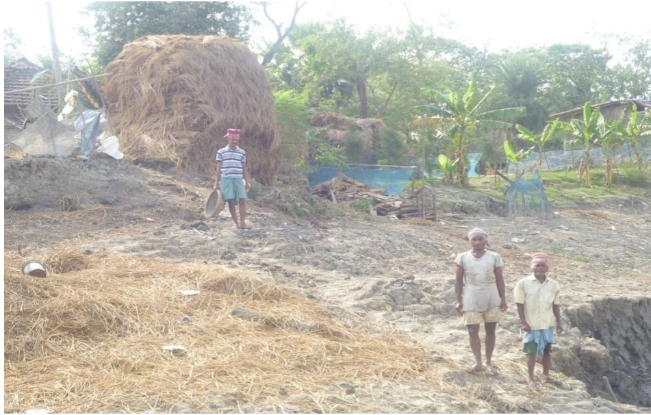
PICTURE-15: RENOVATION WORK AT TETULIA KHAL AT PATHARPRATIMA BLOCK
