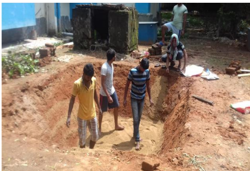
Final semester students digging the stocking pond in outdoor culture unit of the department
