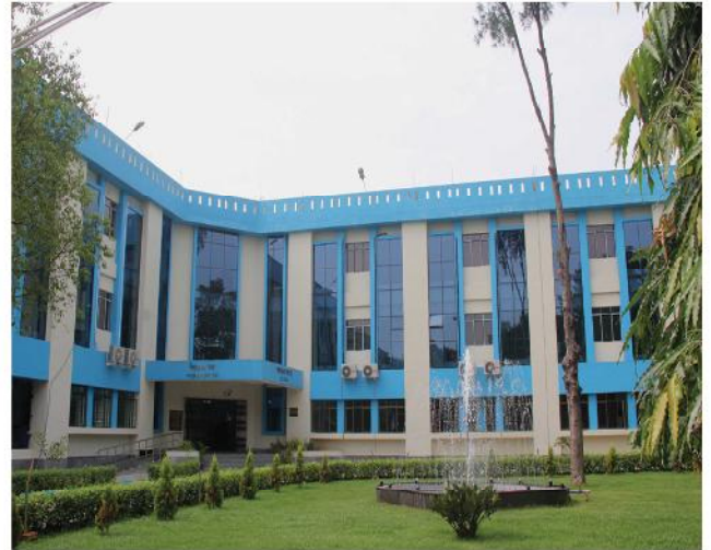
Vidyasagar Bhawan (Annex Administrative Building)
