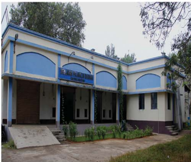
Benjamin Franklin Bhawan (Electrical Substation)
