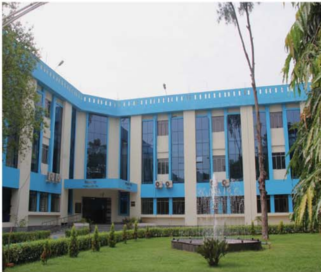
Vidyasagar Bhawan (Annex Administrative Building)
