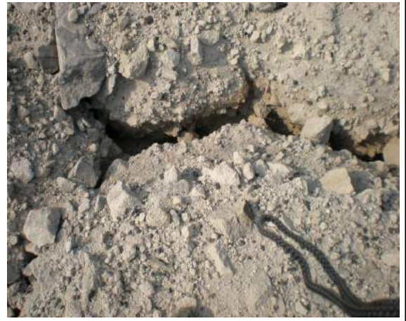
Plate3.3 Cracks on the dumps showing the risk of collapsing due absence of vegetation
