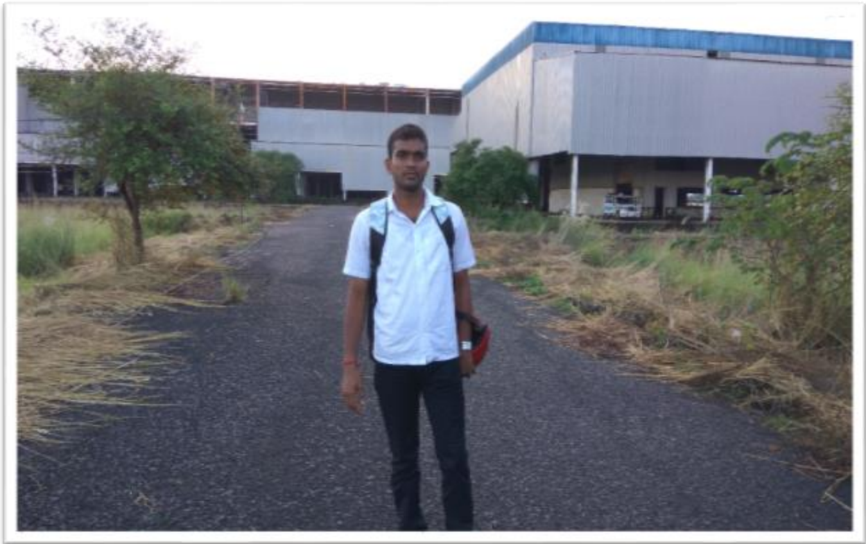
Abandoned structure in Main Workshop inside Tata Small Car Factory, Singur
