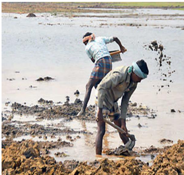
Government worker's restoring agricultural land to its original state in Singur
