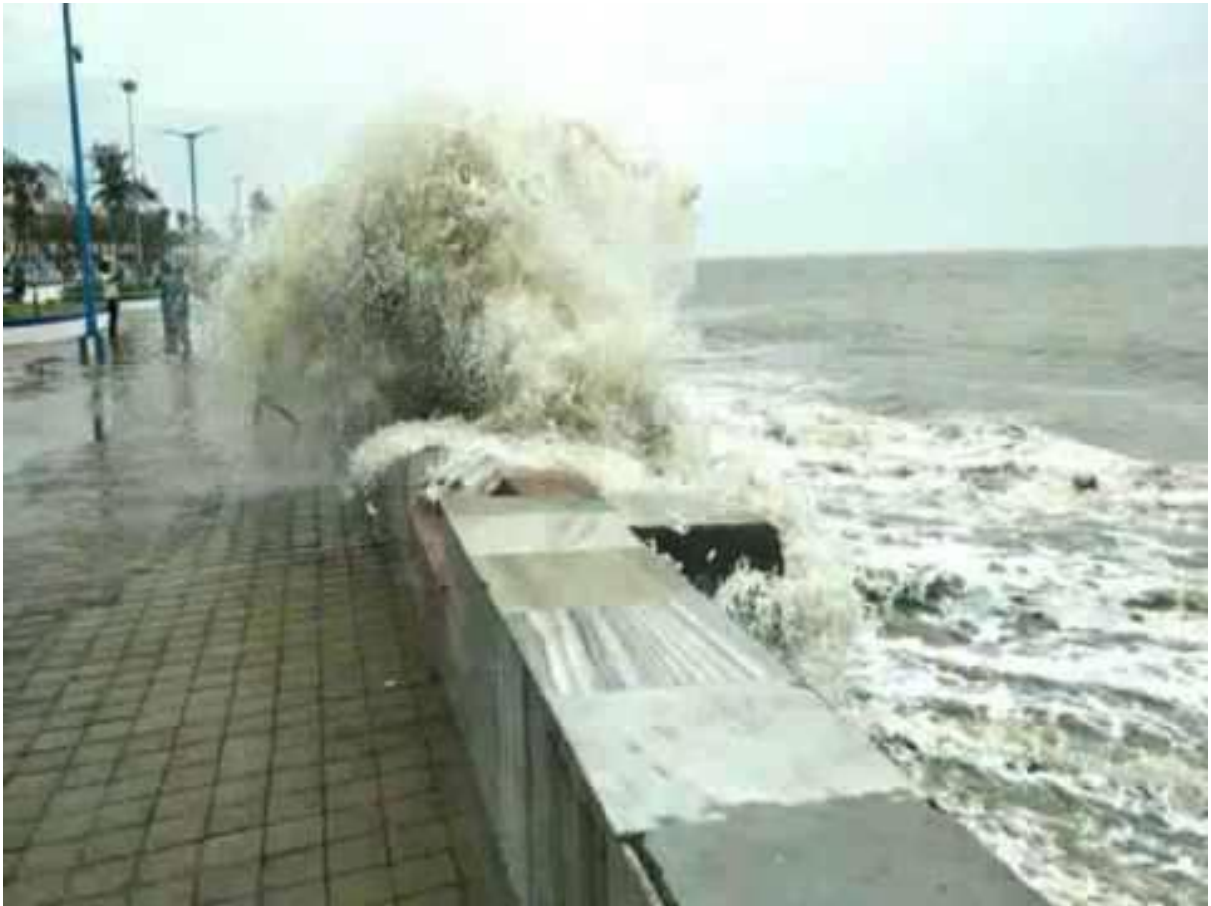
Plate 4.3: Cyclonic storm-wave overtopping the seawall at Digha.
