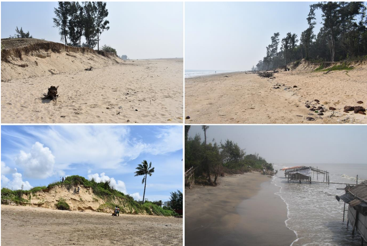
Plate 4.2: Shorefront sand dunes are severely eroded at the different sites of Mandarmani-Sankarpur coastal stretch.
